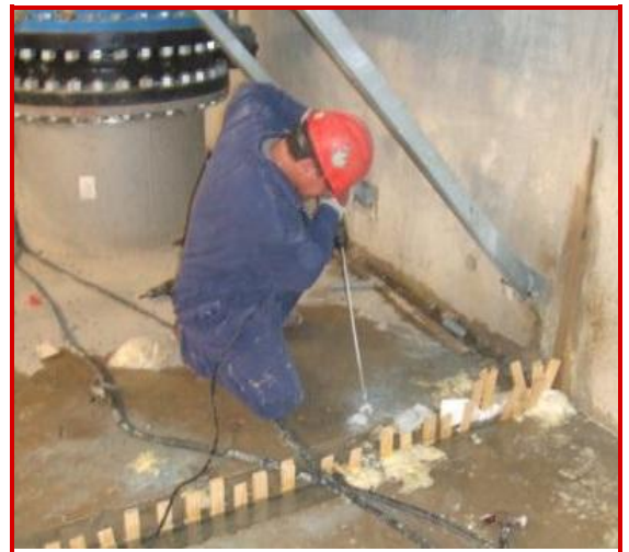
Leaking cracks are permanently repaired using FLEXIBLE RESIN.
