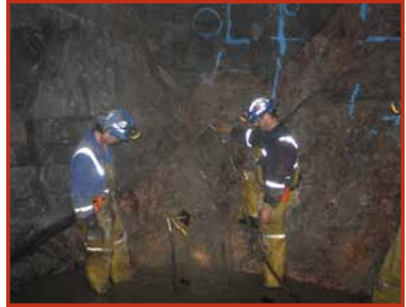
Rio Tinto, Diavik Diamond Mine, Canada Cement grouting methods are used to fill water-bearing fractures and reduce the potential for high-volume groundwater inflows prior to underground mine development operations.
