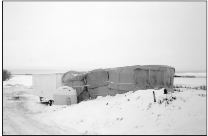
At this cold weather job site, grouting crews were protected from the elements utilizing heated vans and tarps
