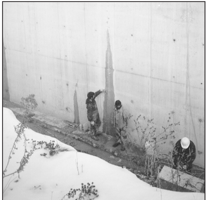
Crews at this potable water reservoir used electric pail heaters to maintain flushing solutions and polyurethane resins at elevated temperatures to combat sub-freezing temperature conditions
