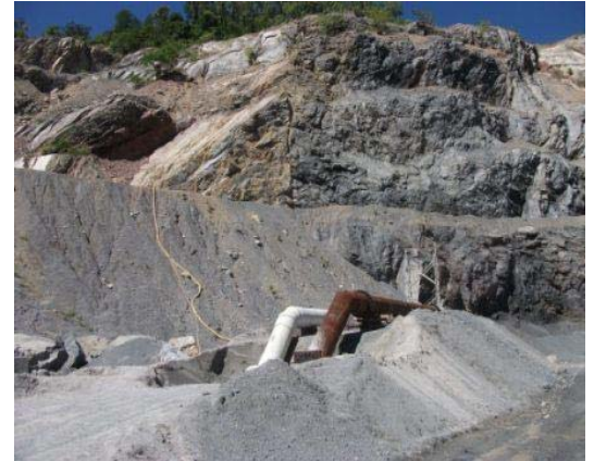
Several full-scale mockups were constructed to observe various aspects of the grouting operation
