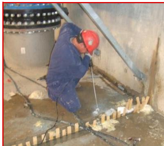
Leaking cracks are permanently repaired using FLEXIBLE RESIN.
