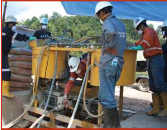
Newcrest Mining, Kencana K2 Project, Indonesia Microfine cement grouts were used to improve ground conditions through fractured and water-bearing ground conditions prior to ventilation shaft construction using raise bore methods.
