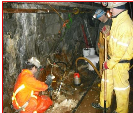
UNIVERSAL RESIN is used to stop water inflow problems for tunneling contractors.
