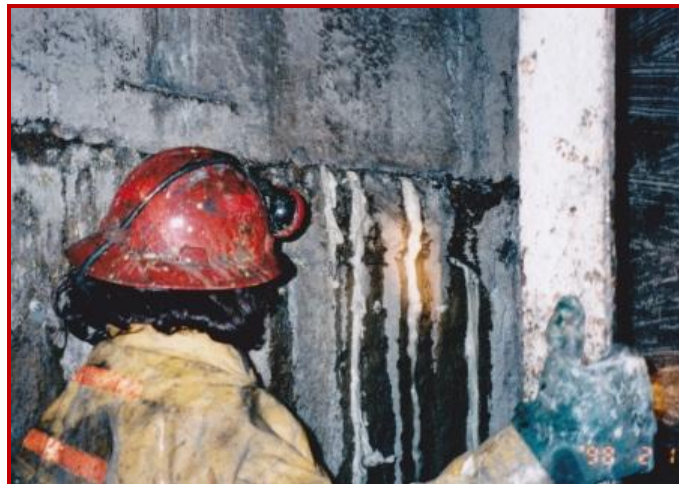
UNIVERSAL RESIN is used to stop water inflows through leaking concrete construction joints in an underground mine shaft.
