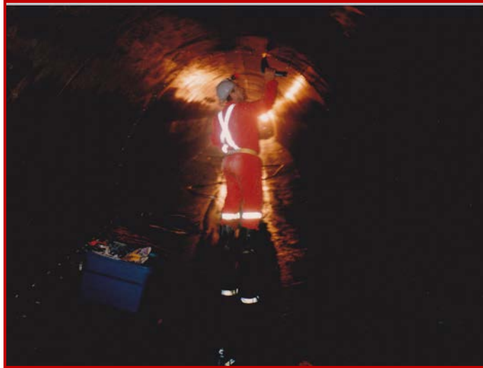
Cracks and construction joints in potable water structures are permanently sealed with MME FLEXIBLE RESIN.
