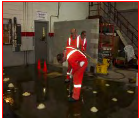
RIGID GROUT is a cost effective solution to fill voids beneath concrete slabs.
