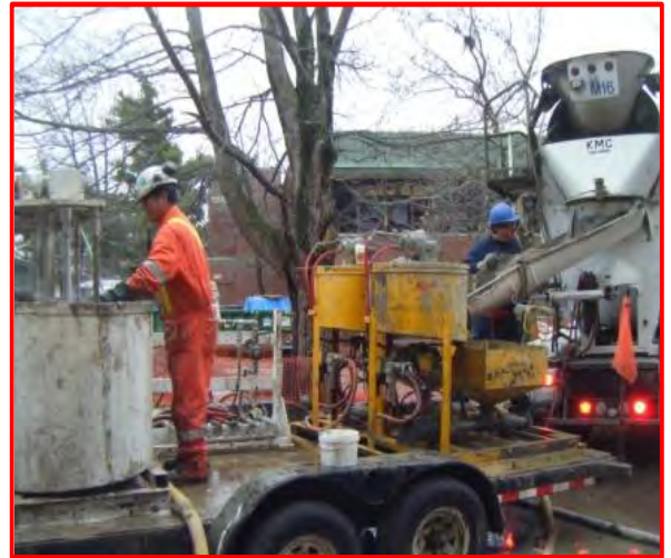
Excavation contractors rely on Multiurethanes' products such as CELBEX 653 to stabilize weak ground conditions.
