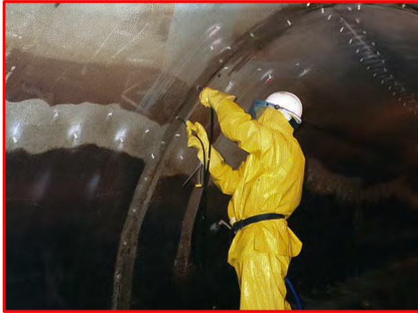
Cracks and construction joints in concrete structures are appropriately cleaned with CRACK FLUSHING AGENT prior to polyurethane injection.
