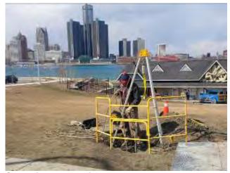
**Chemical Grouting** Windsor, ON Engaged on a chemical grout application based on Universal Resin injection as the appropriate water cut-off solution for a sampling well that intersected a high volume artesian water flow.
