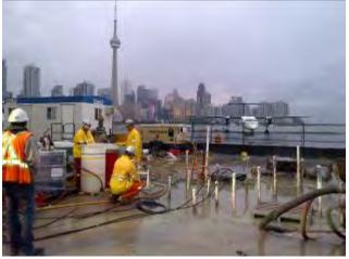
**Soil Stabilization** Toronto, ON Grouting specialist who implemented a soil stabilization grouting program when flowing water was encountered on a pedestrian tunnel construction job site.
