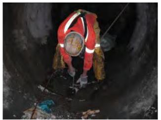
Water Cut off Brampton, ON Engaged on energy transmission facility expansion project performing a water cut off operation in a tunnel shaft liner for a major utility company.
