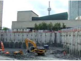
**Soil Stabilization** Toronto, ON Assisted with a chemical grouting operation to stop quicksand from leaking through a caisson wall.
