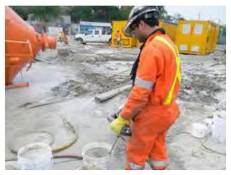
**Cement Grouting** Toronto, ON Performed microfine cement grouting and waterstop operations using polyurethane resins. Provided sodium silicate grouting for soil stabilization in cross passage tunnels in a light rail transit (LRT) line construction project.
