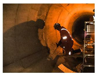
**Cement Grouting to Fill Voids in Tunnel Cross Passage**
