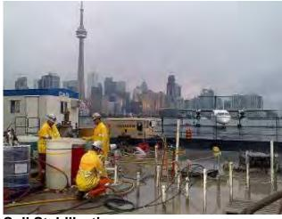
Soil Stabilization Toronto, ON Grouting specialist who implemented a soil stabilization grouting program after surface voids formed during a directional drilling project beneath an airport construction jobsite.
