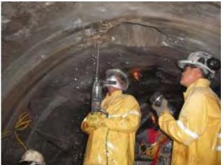
Water Cut-Off Toronto, ON Onsite grouting specialist engaged on a timecritical water stop project to seal active infiltrations through a concrete tunnel liner.
