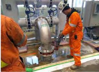
**Hydroelectric Construction** Timmins, ON Performed precision drilling for crack injection work to seal leaking joints and cracks using Universal resin at a hydroelectric generation station.
