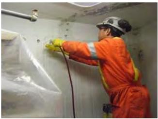
**Chemical Grouting** Brampton, ON Performed strategic polyurethane injection after leaks in underground vaults caused damage to sensitive equipment.
