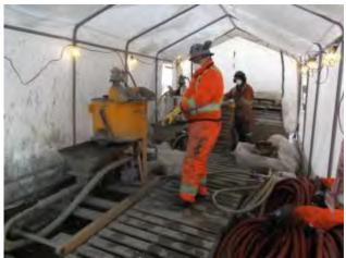
**Cement grouting** Timmins, ON Implemented a grouting program to improve ground conditions in preparation for the excavation of a new ventilation raise by filling existing open rock fractures with cement.
