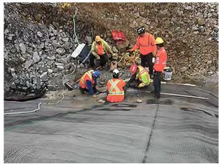
**Consolidation Grouting** Sudbury, ON Performed consolidation grouting and liner welding work for construction of a new tailings dam for a mining company in Northern Ontario.
