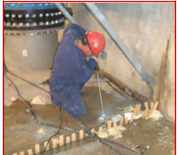
Leaking cracks are permanently repaired using MME FLEXIBLE RESIN.
