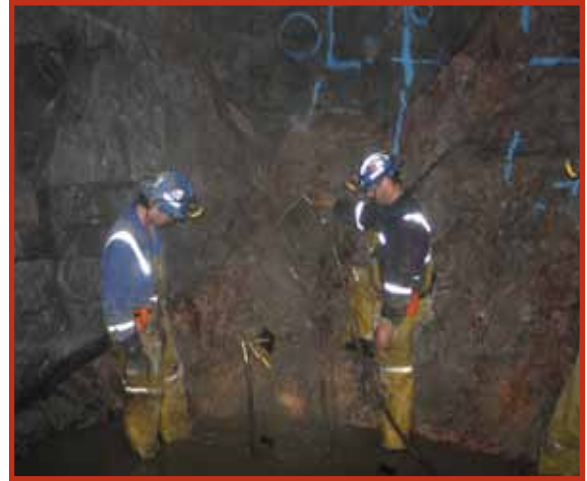
Rio Tinto, Diavik Diamond Mine, Canada Cement grouting methods are used to fill water-bearing fractures and reduce the potential for high-volume groundwater inflows prior to underground mine development operations.
