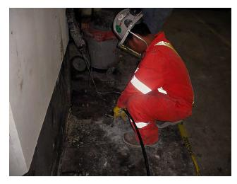
**Chemical Injection in Underground Parking** Burlington, ON Performed chemical grout injection to seal cracks in concrete, preventing infiltration of water through the foundation walls.
