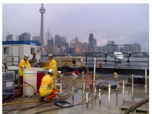
**Soil Stabilization (Toronto, ON)** Implemented a soil stabilization grouting program when flowing water was encountered on a pedestrian tunnel construction job site.
