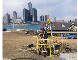
**Chemical Grouting (Windsor, ON)** Engaged in a chemical grout application based on MME Universal Resin injection as the appropriate water cut-off solution for a sampling well that intersected a high-volume artesian water flow.
