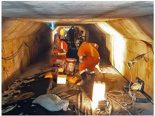
**Crack Injection (Ottawa, ON)** Led a large technical crew that performed chemical pressure grouting in a major culvert repair project that required sealing cracks in more than 600 linear meters under Highway 174.
