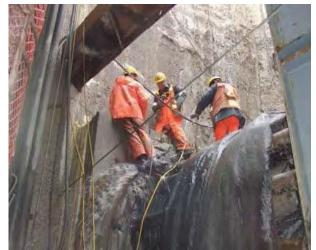
**Cement Grouting (Toronto, ON)** Technical grouting specialist for a shaft and tunnel contractor on a high-volume waterstop project using cement grout, specialty additives and polyurethane grouts.
