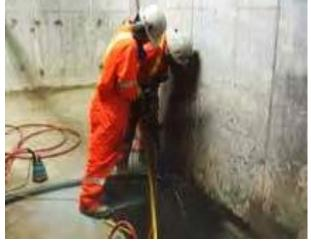
**Void Filling (Toronto, ON)** Provided cement grouting to fill voids and cracks in concrete walls to minimize water migration at a pedestrian tunnel project job site.
