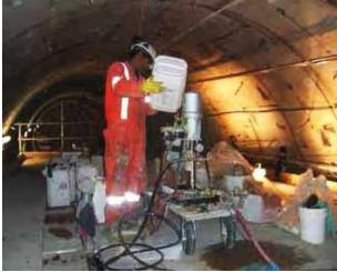
**Tunnel Grouting (Edmonton, AB)** Performed on-time critical sealing of leaking precast concrete tunnel segments using chemical grouts for a large municipal light-rail transit (LRT) system.
