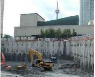
**Soil Stabilization (Toronto, ON)** Assisted with a chemical grouting operation to stop quicksand from leaking through a caisson wall.
