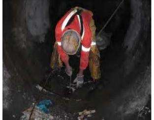
Water Cut-off (Brampton, ON) Engaged in an energy transmission facility expansion project performing a water cut-off operation in a tunnel shaft liner for a major utility company.
