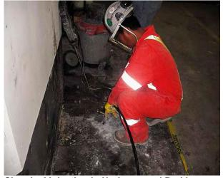
**Chemical Injection in Underground Parking (Burlington, ON)** Performed chemical grout injection to seal cracks in concrete, preventing infiltration of water through the foundation walls.
