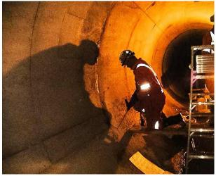
**Cement Grouting to Fill Voids in Tunnel Cross-Passage (Toronto, ON)** Performed cement grout injection to fill voids and stop water infiltration around the cross-passage section in the tunnel.
