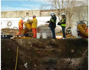
Soil Stabilization Program for Utility Contractors (Toronto, ON) Assisted a utility contractor in the implementation of a soil stabilization program when loose fill was encountered during excavation operations.
