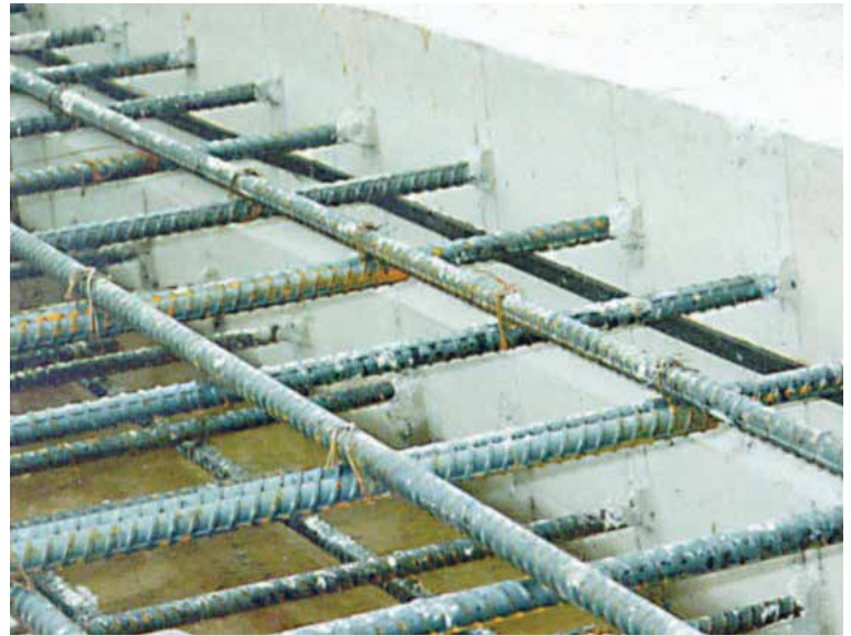
Hydrotite CJ-0725 is commonly installed as a waterstop between new and existing structures during facility expansion projects.
