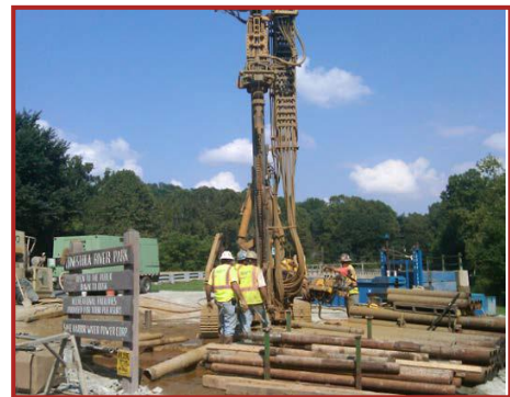
Geotechnical and excavation contractors use specialty additives like CELBEX 653 when working in water-bearing soils to stabilize weak ground conditions.
