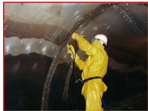
Cracks and construction joints in concrete structures are cleaned with CRACK FLUSHING AGENT before resin injection.
