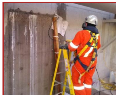
Preparing injection holes for the application of MME FLEXIBLE RESIN to seal active water leaks in concrete.
