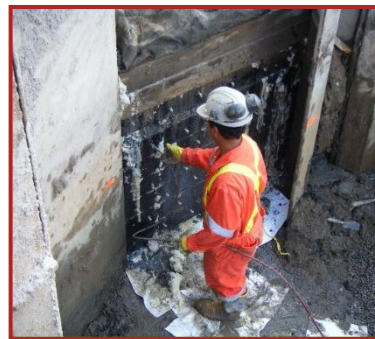
MME Universal Resin stops water inflow problems in deep excavation sites.
