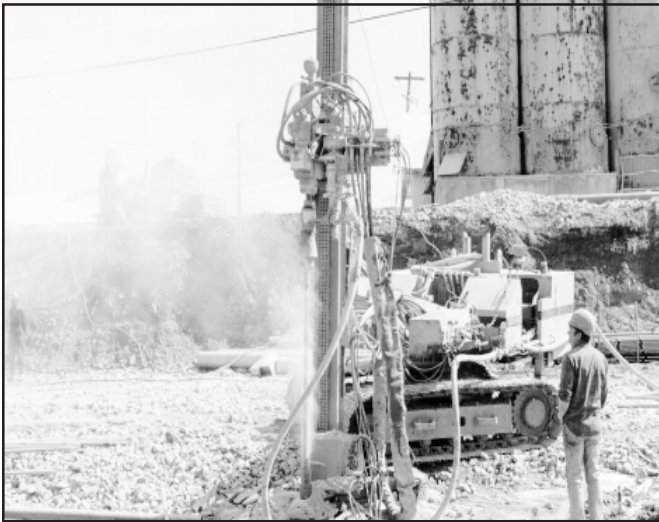
FIGURE 2 - DK 100 Drill Rig in Operation
