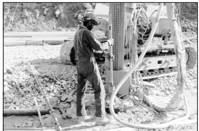
FIGURE 3 - Plastic Sleeve Pipes Being Installed
