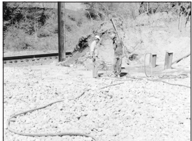
FIGURE 5 - Typical Sleeve Pipe grouting Operation
