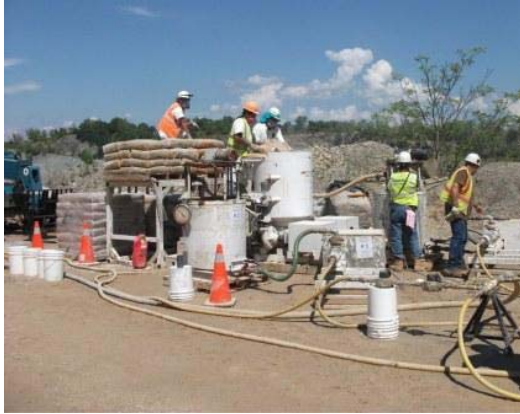
Cement grouting equipment set-up during the trial phase of the project
